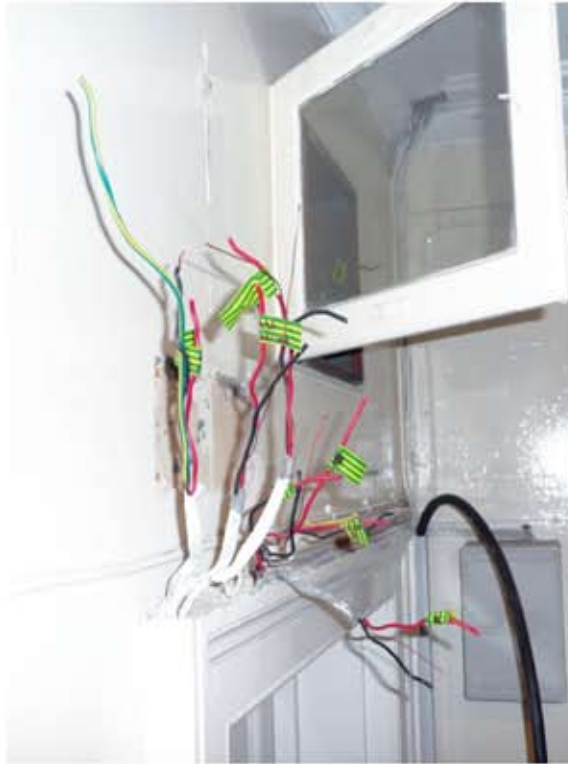
▲ Rewiring – As part of our on-going maintenance and development of the school, we have completely re-wired the buildings and also upgraded the incoming mains supply to allow for future additions to our electronic equipment.
